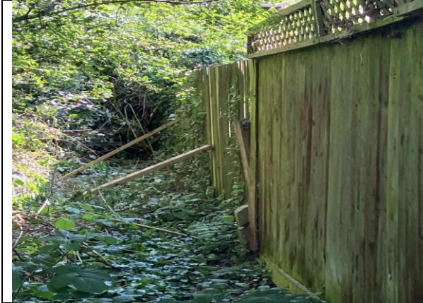
Fence with supports & undergrowth
