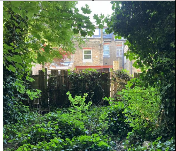
Fence in disrepair
